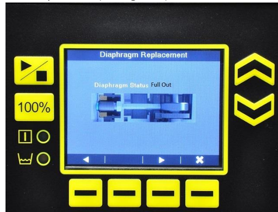
Figure 2 – Full Out diaphragm replacement screen
