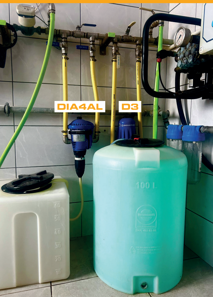
DOSATRON DIA4AL + D3 PUMPS INSTALLED
