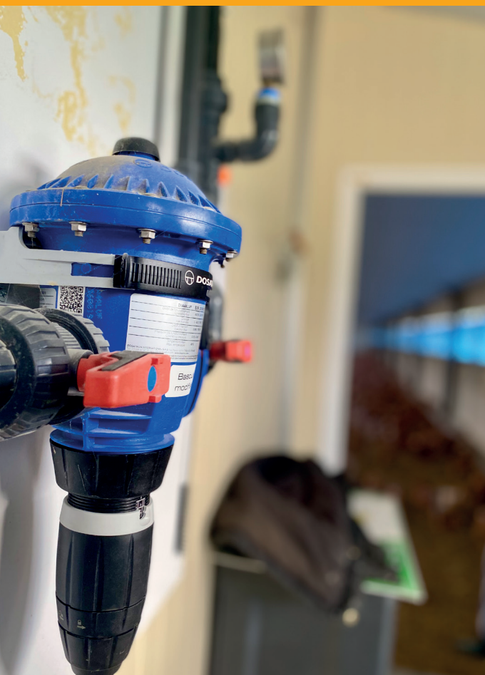
DOSATRON DIA4ALVF INSTALLED
