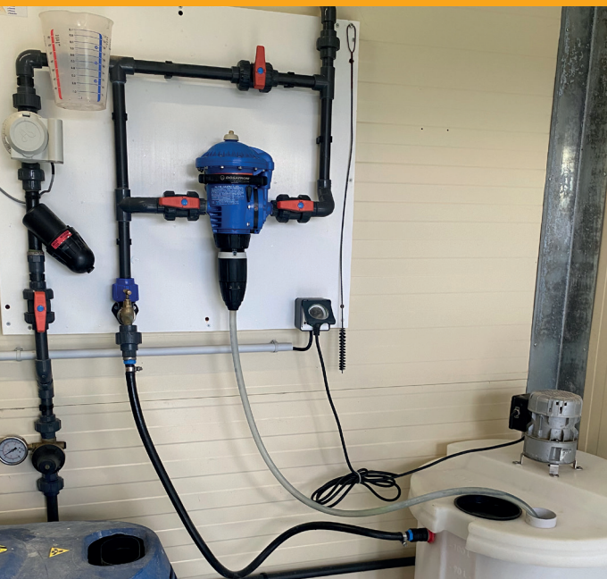
DOSATRON DIA4ALVF INSTALLED
