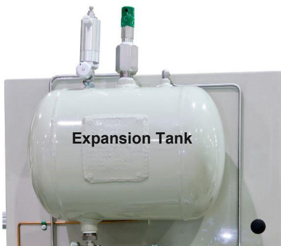
Figure 65 Expansion Tank
