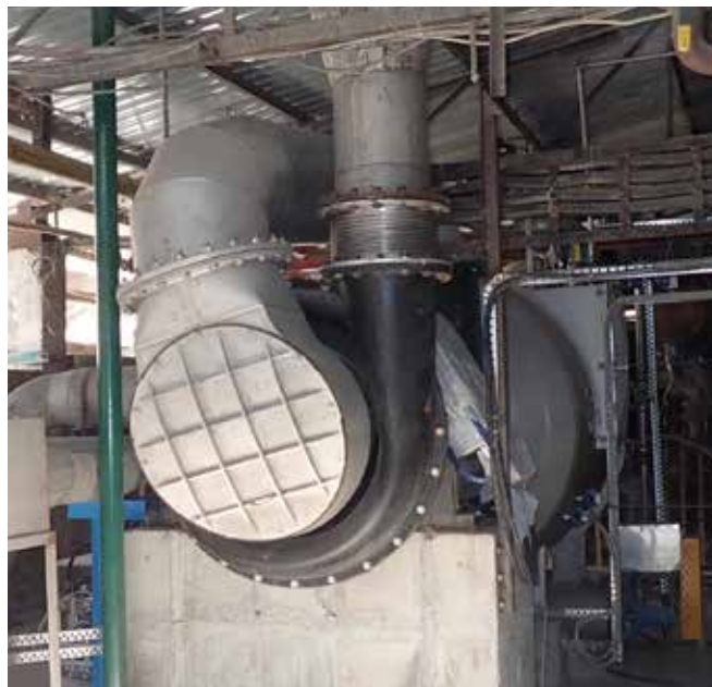
RunEco EP Turbo Blower at Satia Industries Ltd. PM 3.
