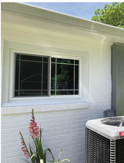
Sliders come in 2- and 3-lite models. 3-Lite Sliders have a center fixed panel and are available in configurations of 1/3-1/3-1/3 and 1/4-1/2-1/4 .
