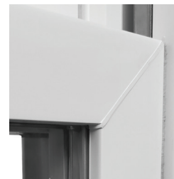
Fusion-welded corners prevent air from passing through and boost structural support.
