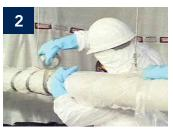
If the insulation is friable, wrap the pipe with a layer of polyethylene sheeting with duct tape in a "candy-stripe" pattern.
