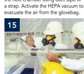
Remove all of the glovebag work area stubs remaining, starting at the collar, slitting the top of the stubs free while folding inward into an asbestos disposal bag.
