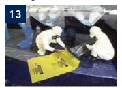
Place the debris chamber into a properly marked asbestos disposal bag and move on to the next chamber and repeat the process.
