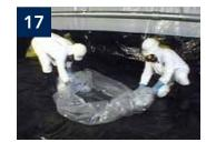
After the last chamber of the Extended-Run Glovebag has been taken down and safely disposed of, proceed with clean up and decontamination.
