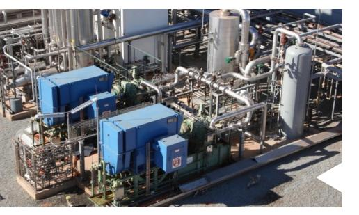
Online since 2007, Ingersoll Rand integrally geared compressors provide reliable refrigeration at this LNG plant
