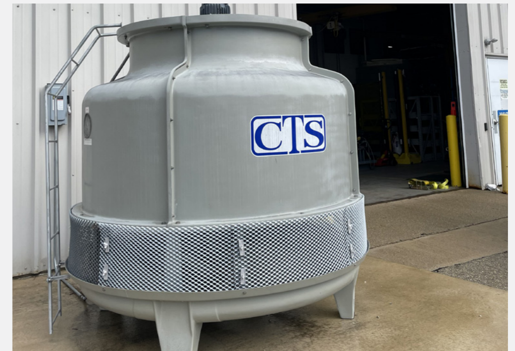
Enon, Ohio site: Cooling tower for R&D test bench
