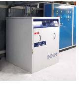
A famous pasta maker installed Robox Screw for flour and sugar pneumatic transport due to its lower temperature operation, lack of deterioration of the conveyed material and high energy performance.
