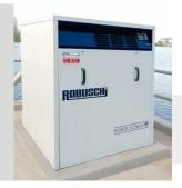
The customer decided to install Robox Screw in order to provide a curtain of air bubbles to prevent floating and submerged objects from entering the docking area. They are impressed by the unit's robustness and heavyduty capabilities.
