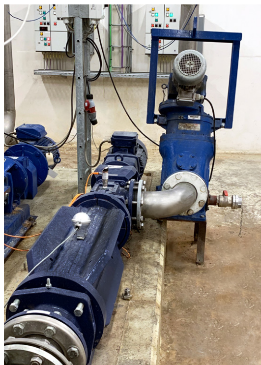
BN 52-12S SCT with Pump Monitor sensors at the Lynetten treatment plant.
