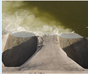
Gilbert Road Pipeline
