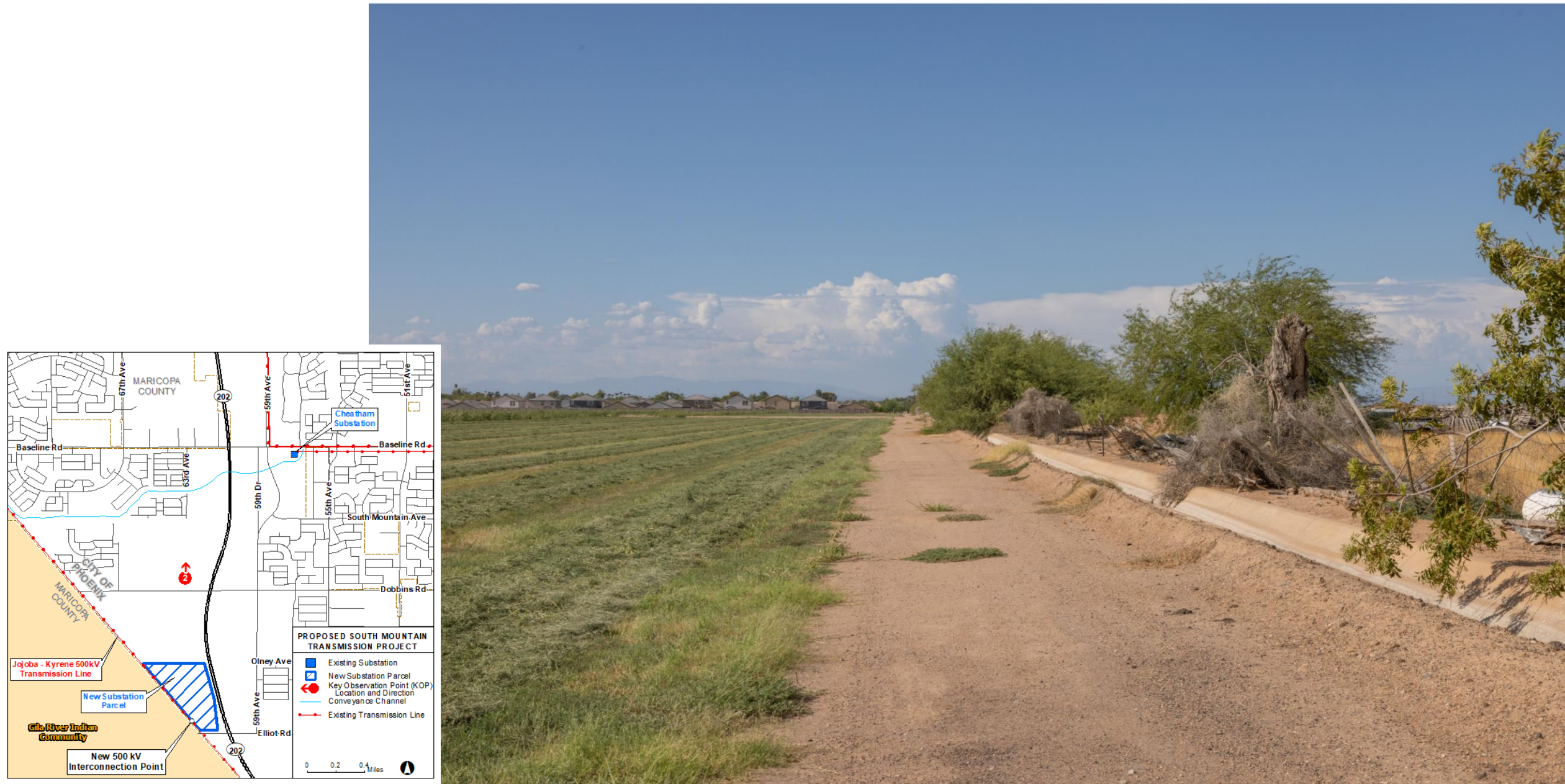
Existing Conditions South 63 rd Avenue Looking North
