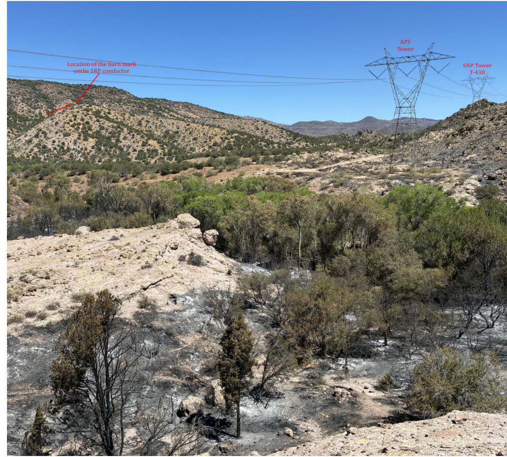
Gold Fire: 500kV Coronado-Silver King line. Red arrow shows the SRP conductor is lower than the APS conductor in the foreground. No damage resulted from the wildfire
