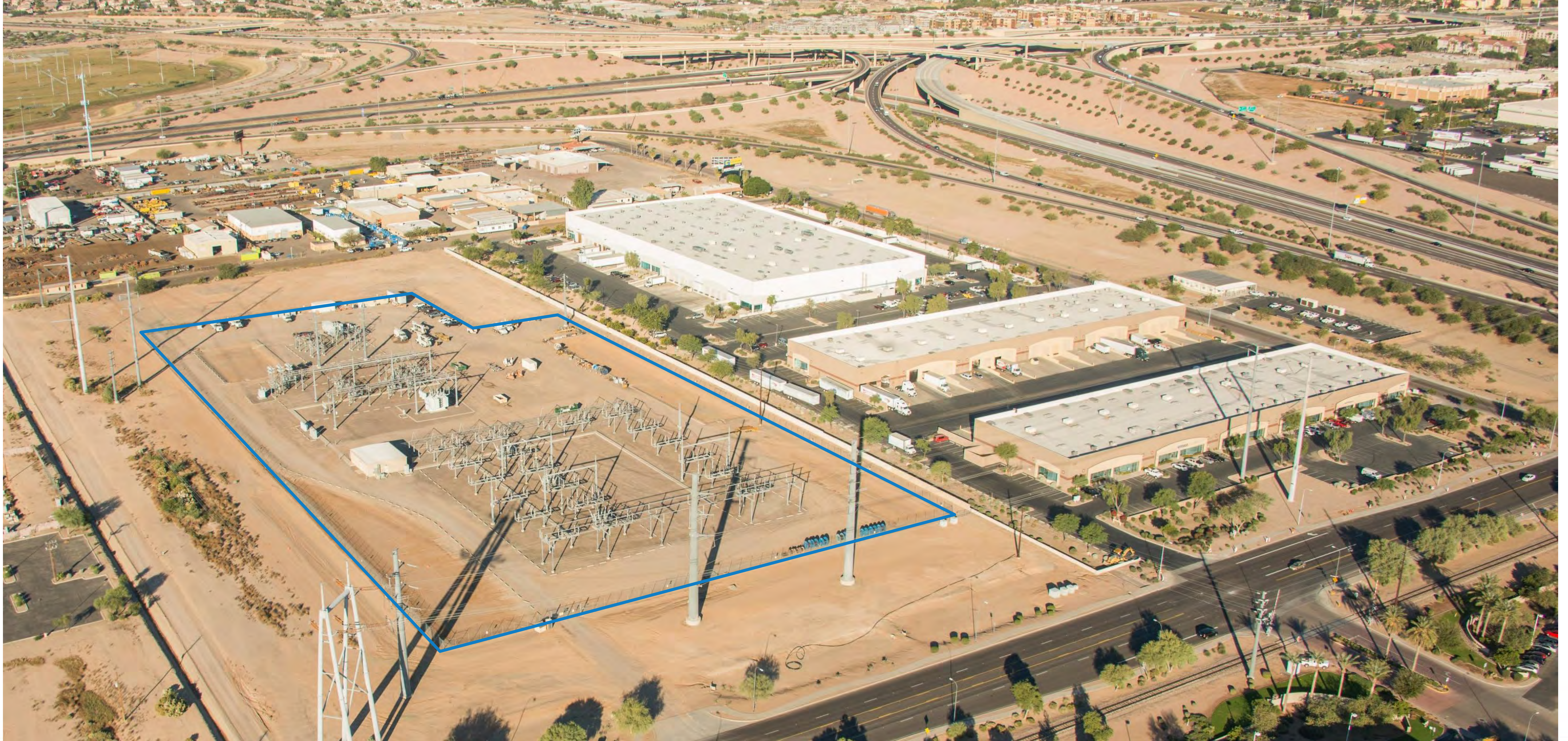
Typical 230kV Substation
