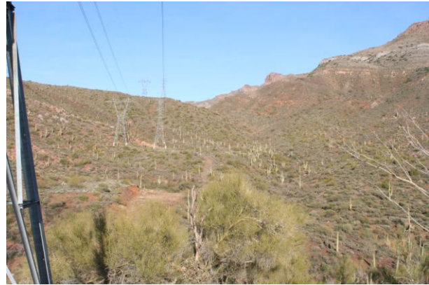
Photograph 2. View of the existing 230kV and 500kV transmission lines in the vicinity of Silver King Mine Road.
