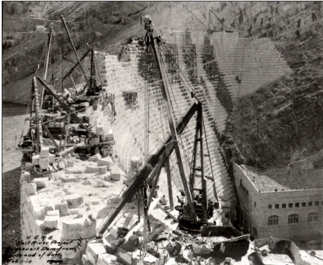
Roosevelt Dam construction, stiff legged derrick, 1910
