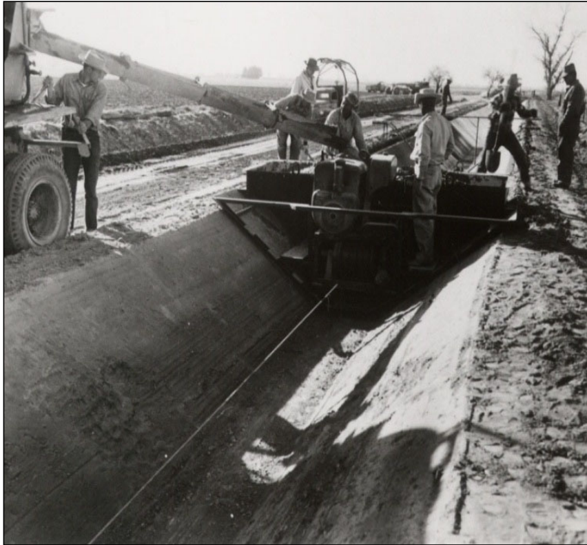
Slipforming lateral, c. 1960
