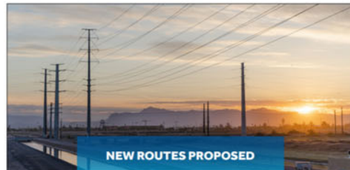
New transmission lines and substation
