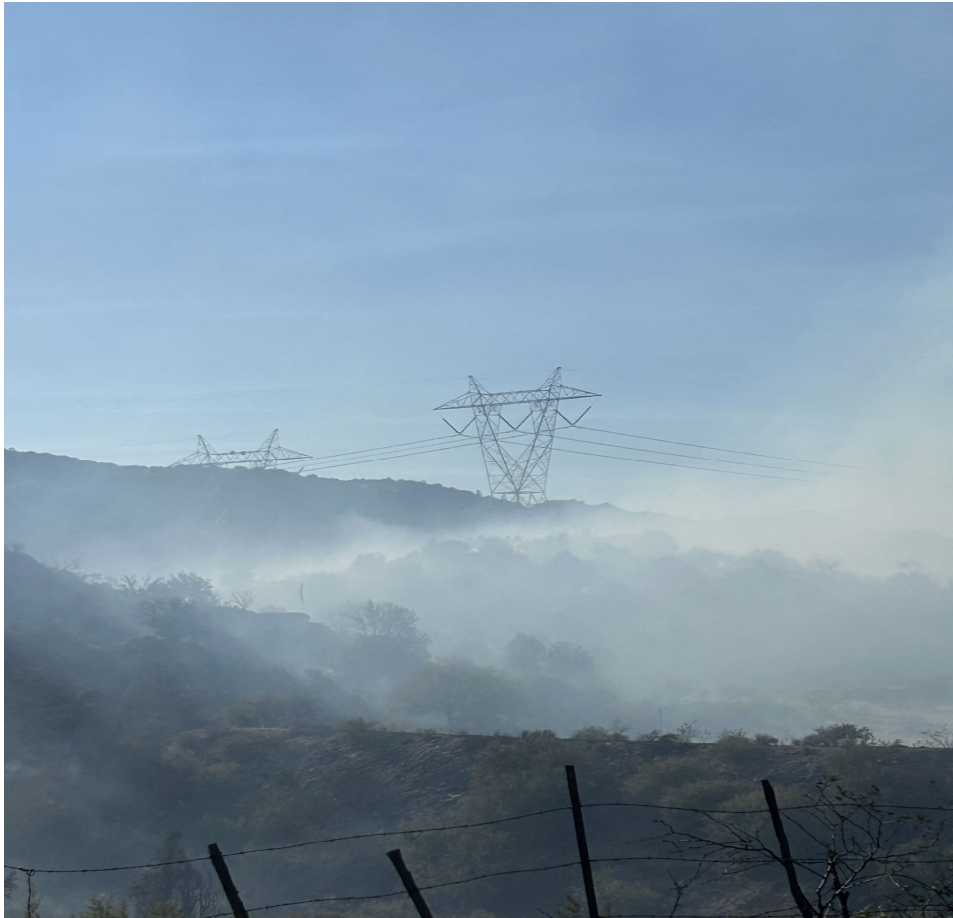
Gold Fire: White smoke from the fire on June 27, 2026, as it moved through riparian vegetation northwest of Pinto Valley Mine (northwest of Miami, AZ)
